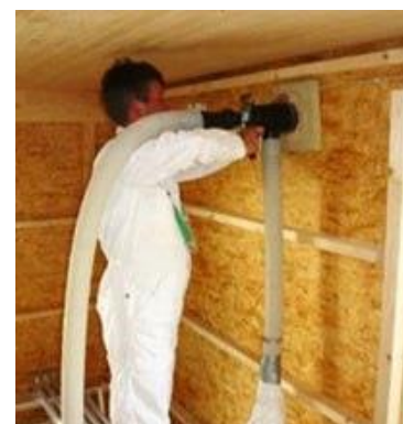
Figure 4: Cellulose insulation in a wall
