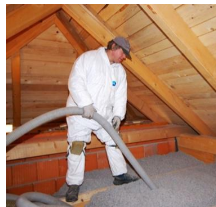
Figure 2: Cellulose insulation in open attics
